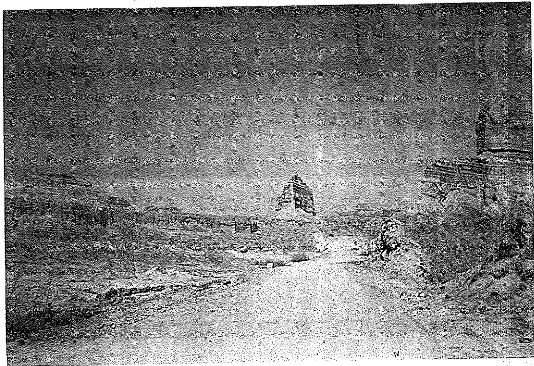
Photograph - 13 Road passing through clayey mountain in section-2
