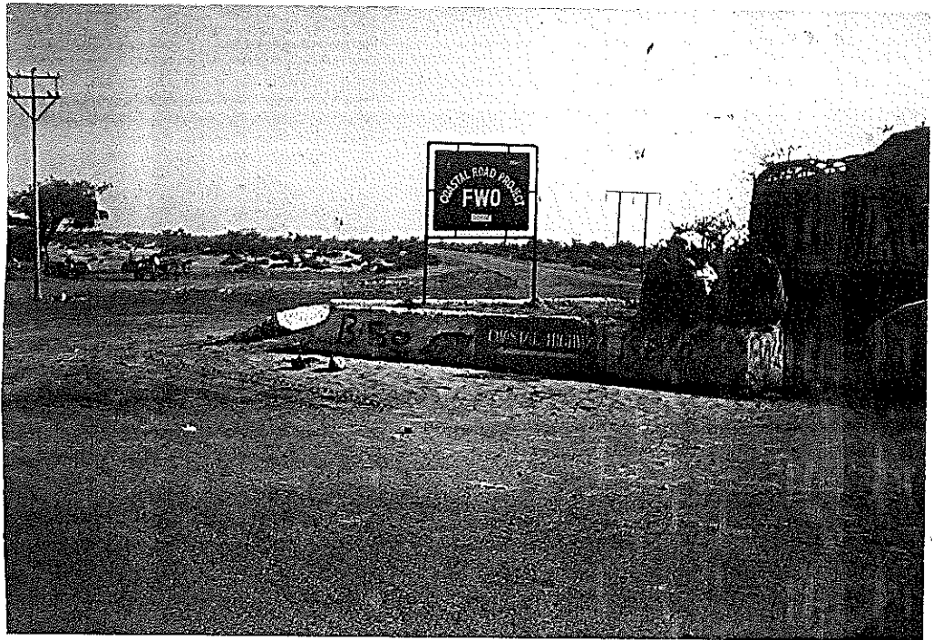
Photograph - 1 Zero Point of Coastal Highway at N-25
